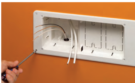
1 Install NM94 cable connector, and power and low voltage cables.
