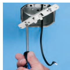
1 Attach SC5 bracket to box.
