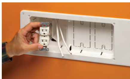
3 Install power and low voltage wiring devices.
